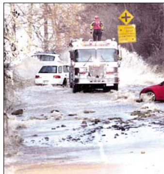
A rupture in a 66-inch pipe flooded Bethesda's River Road in December.
